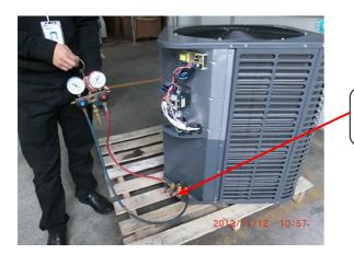
Connect the high and low pressure gauge to outdoor unit
