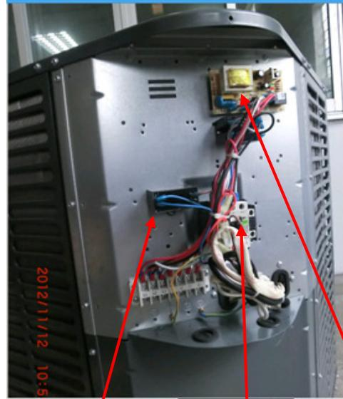
Fan capacitor      Contactor      Phase sequence board
