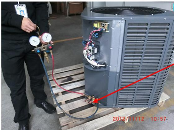
Connect the high and low pressure gauge to outdoor unit
